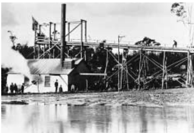
Water sluice at Echunga, erected in 1907 to rework the large Jupiter Creek alluvial goldfield. Alluvial gravel was placed at the top of the sluice and washed over corrugated riffles where gold collected. (Photo 24062)
